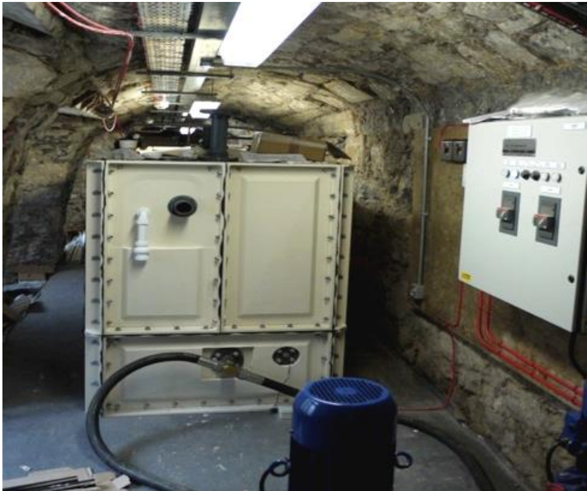
16thC masonry vault with 6m 3 modular Water Storage tank offering 30 minutes water mist system coverage. Photo Stewart Kidd
