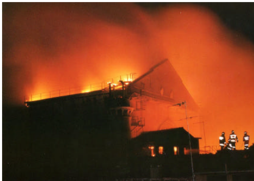
Photo n. 1 - In the night between 12 and 13 December 1996 a fire destroyed great part of the Great Theatre "The Fenice", in Venice. In this case a temporary alteration caused by the construction site has contributed to spread fire and hindered the operations of firemen teams'.
