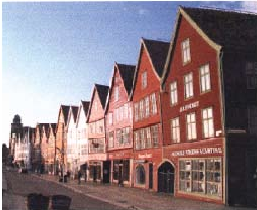
Bergen Wooden Town protected by Gornner System
