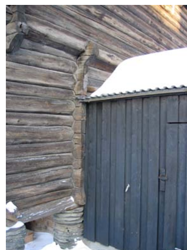
Fire engine high pressure pump connection (middle of dark wall) to flashover suppression system (Marioff, Hi-fog) in historic mining town Røros. Pic: G Jensen.
