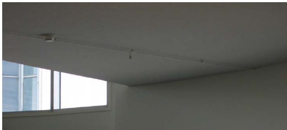
Hi-fog nozzles, welded to pipe. To the right, painted white
